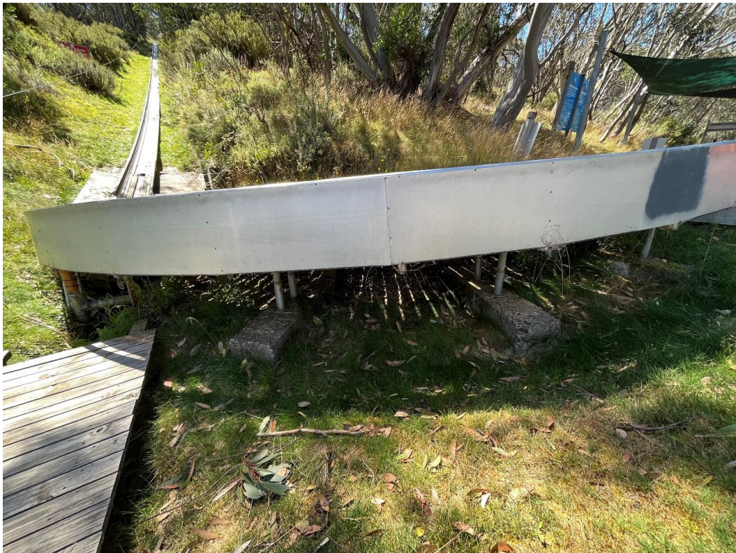
Photo 4 – supports for first curve before cable run, not shallow concrete footings
